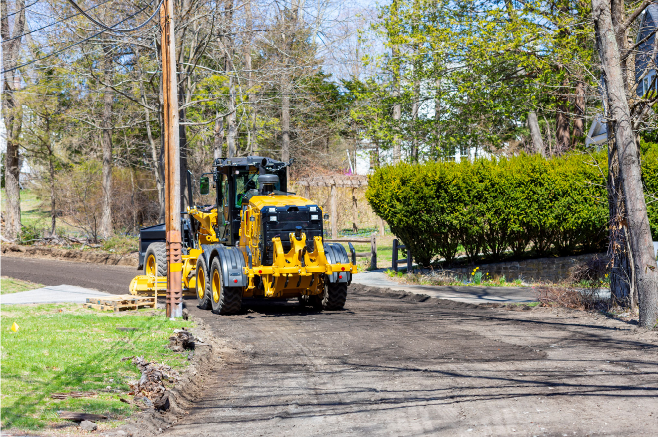
Photo above: Richard Street paving.
